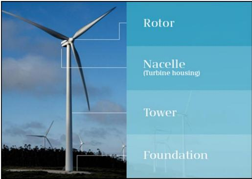
Plate 2-1 Wind turbine components
